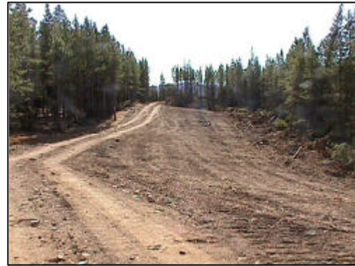
Newly constructed fireguard – Venables Fire, near Ashcroft
