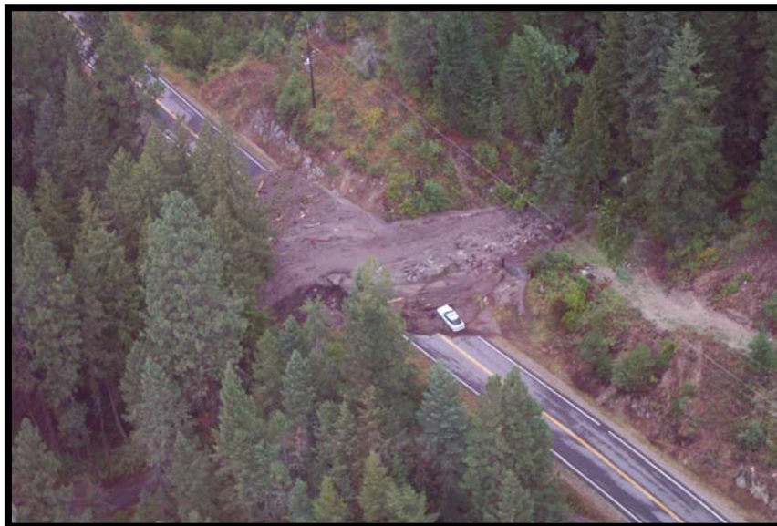
Debris flow on Highway 3A at Jansen Creek, August 7, 2004.
