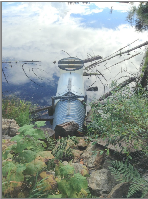
Figure 17. September 17, 2013 – The beaver proof culvert inlet.
