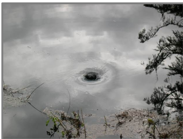
Figure 4. May 27, 2004 – The culvert inlet has been unplugged and the lake is draining.
