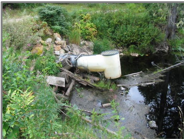
Figure 10. August 21, 2012 – The beaver proof add-on is not seated properly. The original, lower culvert is obscured by debris. Some of the blocks of wood that can be seen floating in Figure 8, taken two years earlier, now appear to be restricting the lower culvert. Cooke Creek FSR is visible in the top left.
