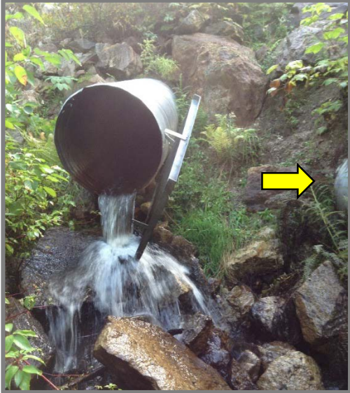
Figure 18. September 17, 2013 – The beaver proof culvert outlet. The original, lower culvert is just visible to the right, indicated by the arrow.
