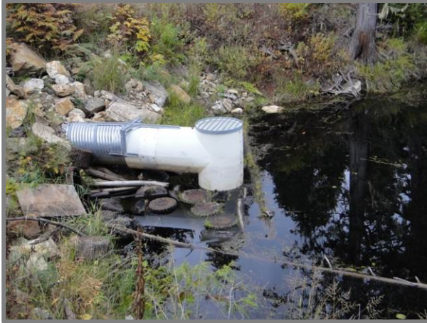
Figure 8. October 11, 2010 – The beaver proof add-on attached to the culvert inlet. The original, lower culvert is just visible behind the rectangular piece of material, (possibly plywood). Note the floating blocks of wood.
