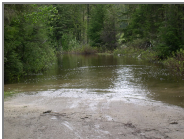
Figure 3. May 27, 2004 – Water from Dale Lake overtopping the Cooke Creek FSR at the 8.5-kilometre point.
