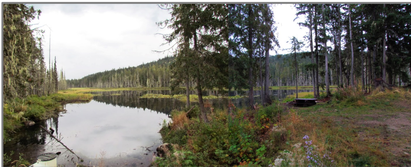
Figure 1. The Dale Lake recreation site on September 25, 2011. The top of a beaver proof culvert is visible in the lower left.
