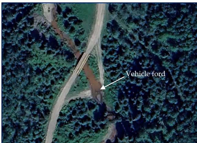
Figure 3. Google Earth image showing the bridge structure and vehicle ford on Bernadet Creek.
