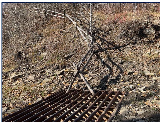
Figure 5. These range developments, including a post and rail fence, and a cattle guard, are in an effective operating condition.
