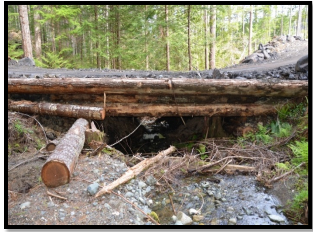
Bridge located at the bottom of a hill, on a curve and there are no guard rails. Superstructure was not lashed or pinned properly to the foundations. No consideration for unbalanced loads or off-centre driving. This bridge was examined during a 2013 audit.
