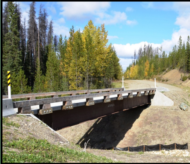
A well-constructed bridge.
