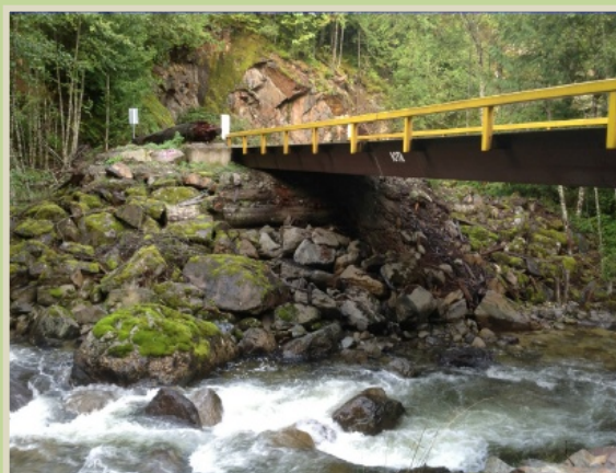
This bridge was designed and built to pass the peak flow expected every 100 years.
