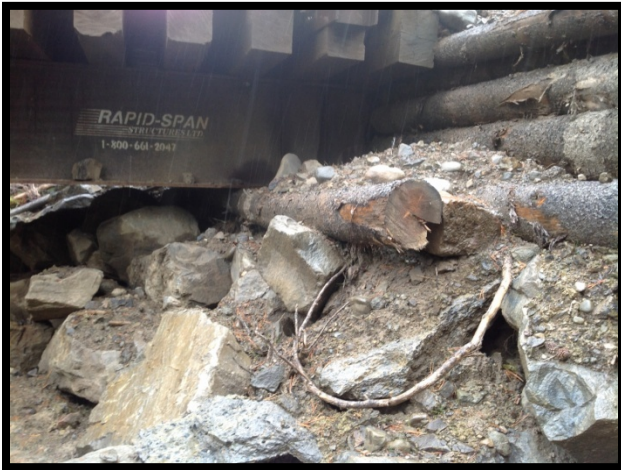
Undersized and improperly located sill log does not adequately support superstructure. Girder stiffener and bearing plate does not align with center of sill
