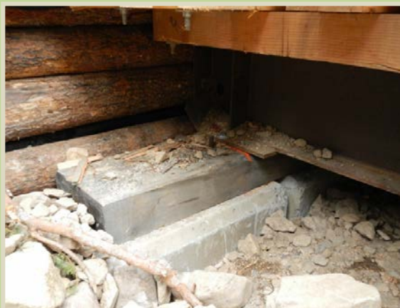
The steel superstructure is bolted to the timber cap and the deck panels are properly attached.
