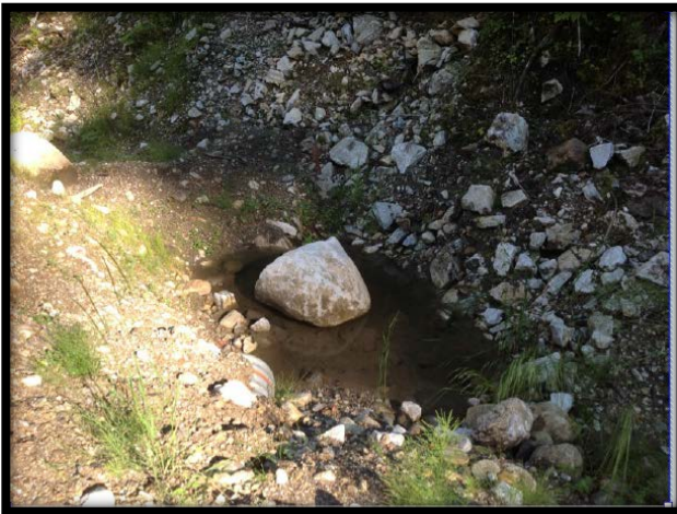
Good sediment control. This sump allows sediment to settle out of the water.
